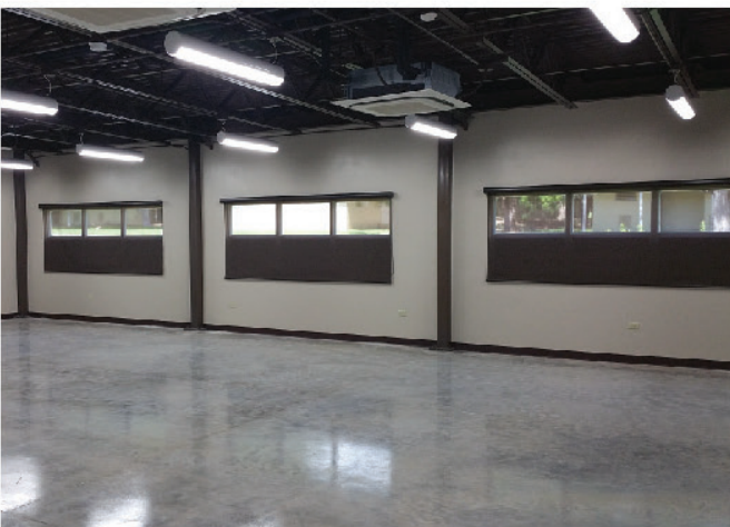
MODERNIZATION OF DORMITORY BUILDING 414
